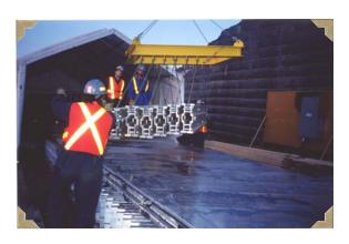
Sectional model LHK12D 312112 is comprised 12 platen sets covering a platen area of 312" x 112" ( 7924 mm x 2845 mm) with a splice length of 285" (7256 mm). Operating pressure for this 94" (2400 mm) wide ST7000 belt is 200 psi  $(14 \text{ kg/cm}^2).$
