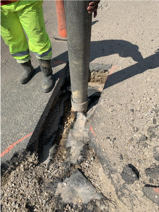
Close-up of vacuum excavation probe. After utility is located and surveyed, the hole is grouted and patched to match existing conditions
