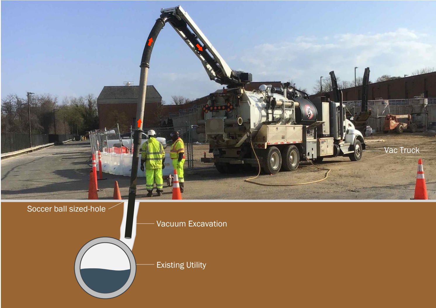
Close-up of vacuum excavation probe. After utility is located and surveyed, the hole is grouted and patched to match existing conditions
